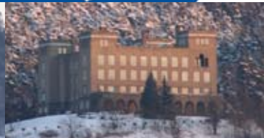
9 Former Maritime School Built 1917
