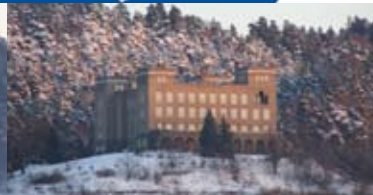
9 Former Maritime School Built 1917
